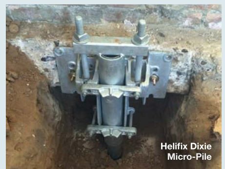
Helifix Dixie Micro-Pile installation
